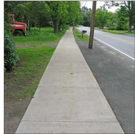
Looking towards Cross St
