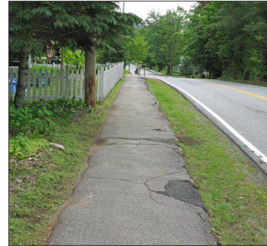
Looking towards Cross St
