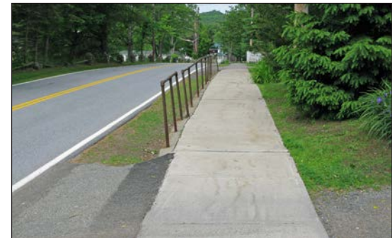
Section of handrail alongside sidewalk
