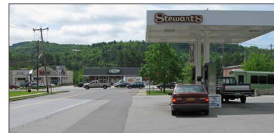
Sidewalk has been paved over in front of gas station
