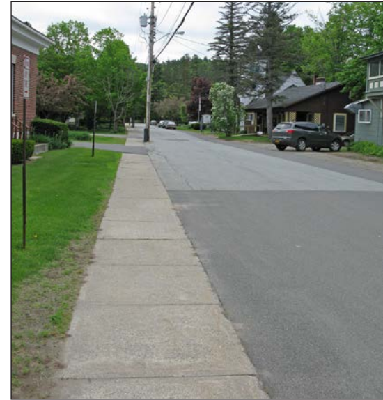
Looking towards Hand Ave
