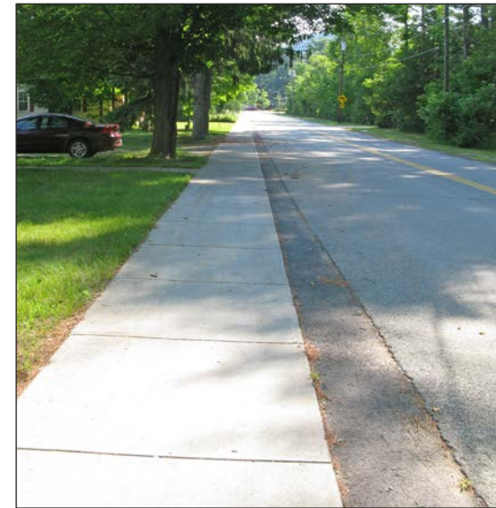
Looking from Williams St toward corner
