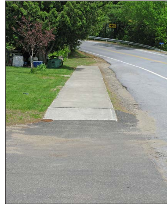
The sidewalk segment northwest of Evans St
