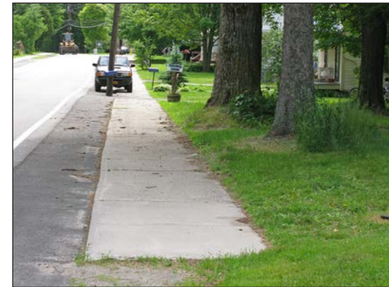
Looking at the end of the sidewalk
