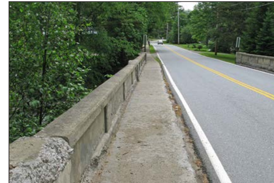
Sidewalk over the bridge
