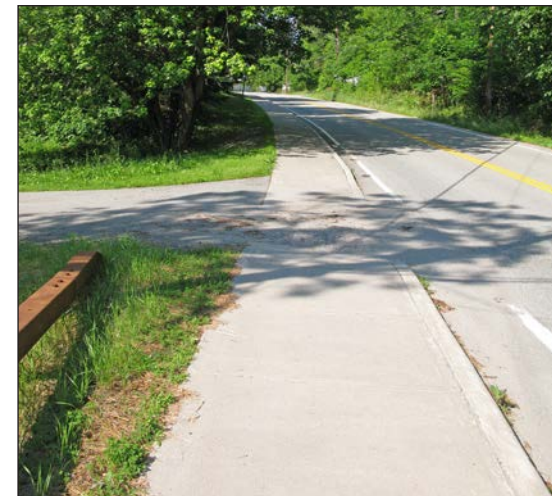
Looking southwest from bridge
