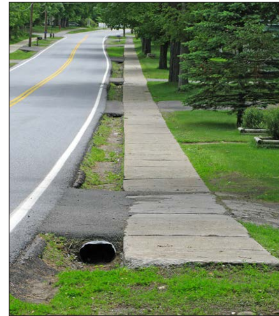
Looking from end of sidewalk east towards Foot Bridge Ln
