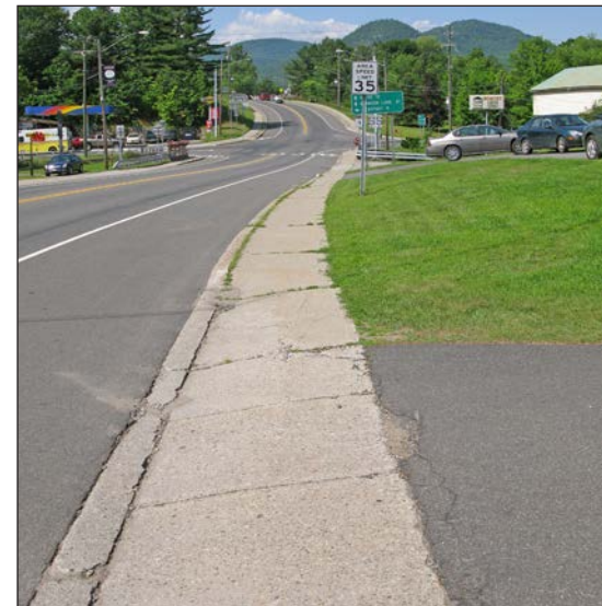
Looking towards the Water St intersection
