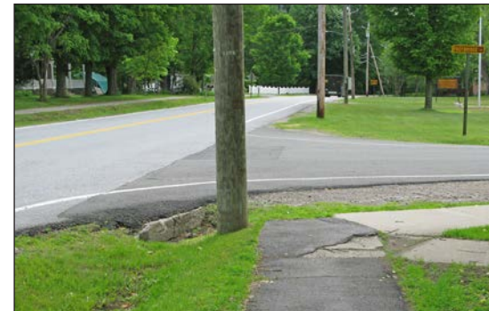
Looking across intersection of Foot Bridge Ln
