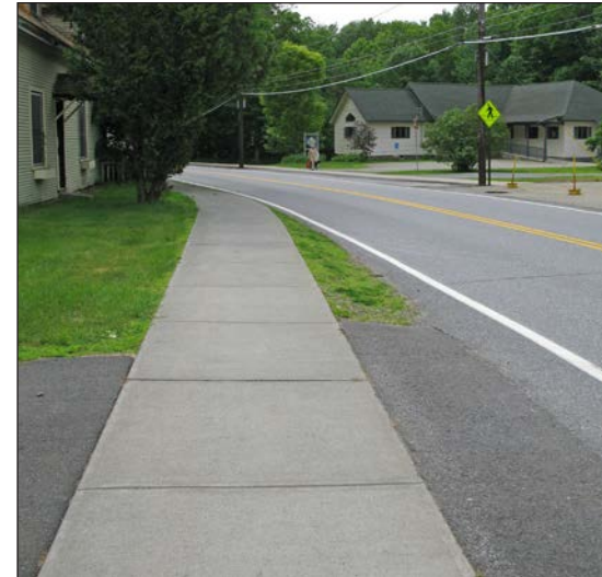
Looking towards Noble Ter along sidewalk across from post office
