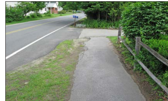
Sidewalk ends at driveway
