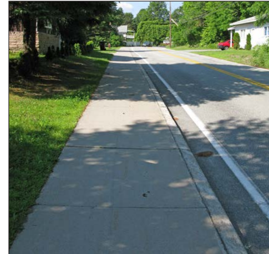
Looking towards the Maple St intersection
