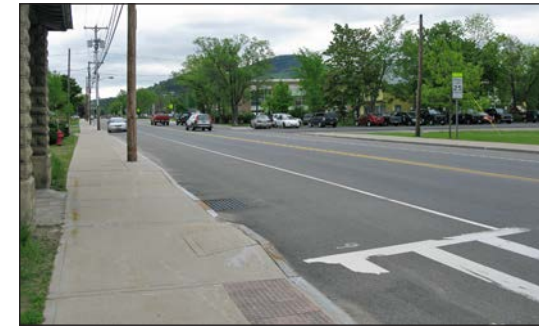
Curb at the Court Street crosswalk
