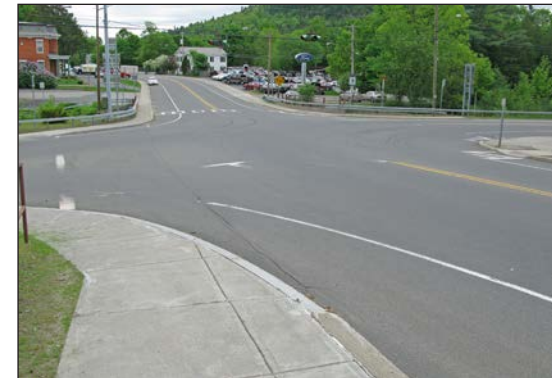
Looking across intersection from Court St towards Maple St
